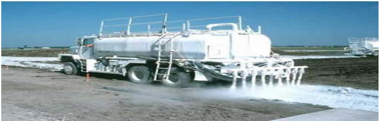
Fig. 3 Spreading of lime over scarified soil
