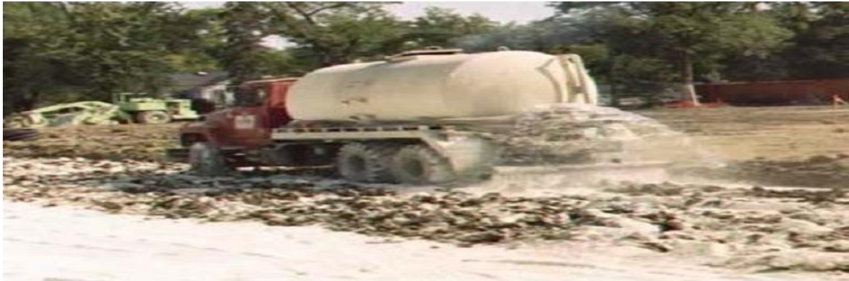
Fig.4 Adding water after dry lime application
