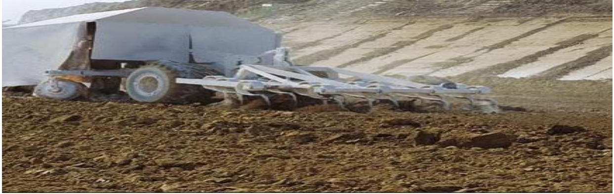
Fig. 2 Scarification before lime application
