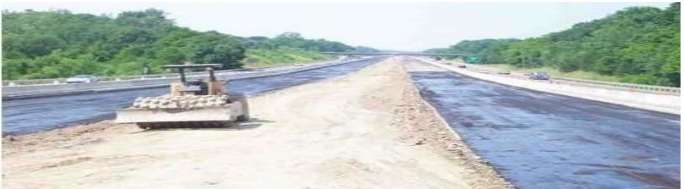
Fig. 7 Prime coat emulsion for curing
